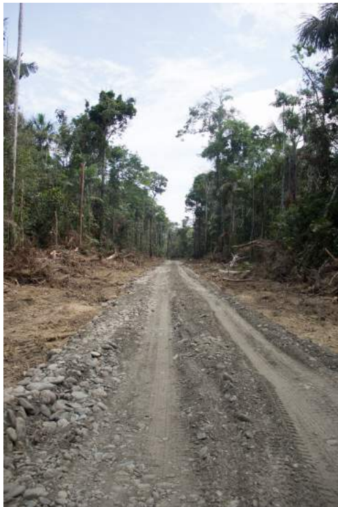
Fig. 3 Progress in the construction of the Manu Road (September 2015). The photograph represents a typical section of the Manu Road, which is made up of a gravel road surface extracted from the nearby riverbed. The cleared areas can be distinguished from the surrounding undisturbed rainforest
